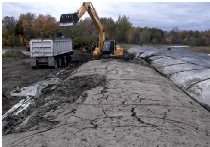
Figur 6-8: Sediment afvandet i afvandingsposer
