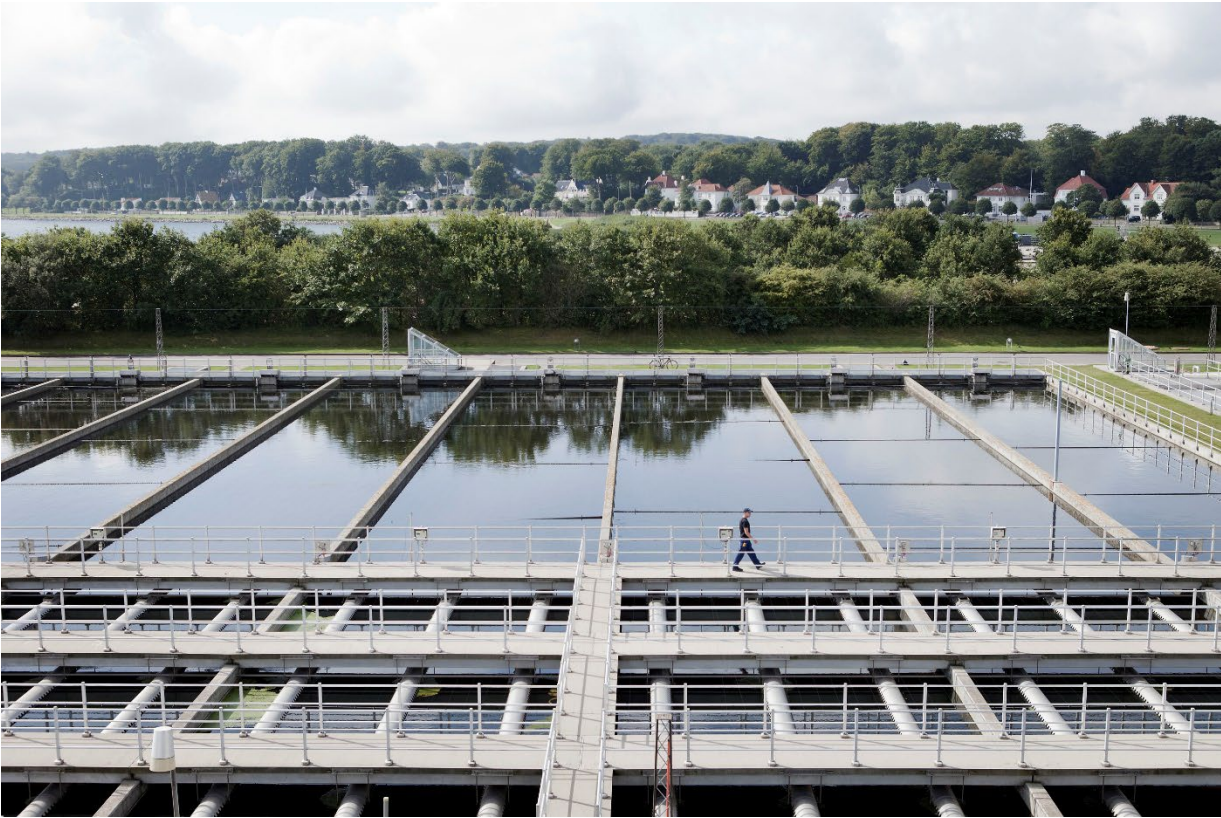
Photo: Marselisborg WWTP, Aarhus
